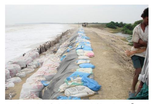
Fig.2 Erosion in the seaward side of Embankment at Pentha (Photo taken on 15<sup>th</sup> November 2007)
